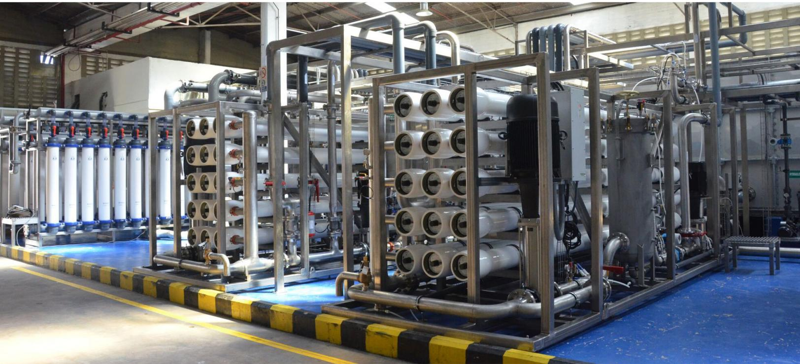
*Demand for water is high and global resources are limited. Reverse osmosis (RO) is an effective and widely-applied water treatment purification method, yet current RO systems waste both water and energy. This paper discusses how RO water treatment can be improved with closed circuit or semi-batch RO techniques. These processes increase water use efficiency, reduce energy consumption, increase flexibility and reliability,*
